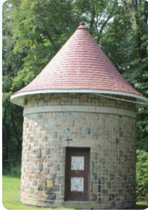
Renovations were completed on valve house at Torrance Tank.
